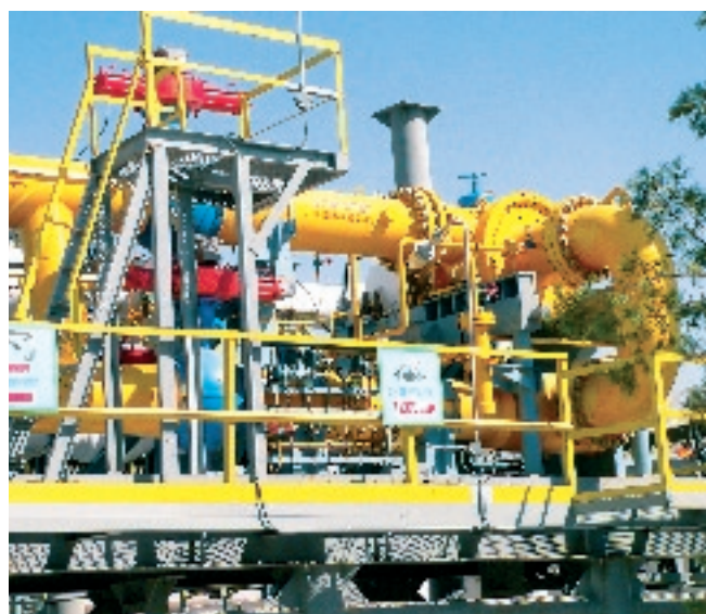
| photo 11 | MTDA – 9,0 – 4,5 – U1 (Republic of Uzbekistan)
